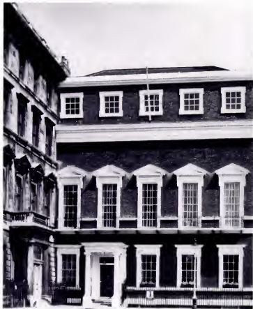
FIGURE 10. No. 4 St. James Square. The duke of Kent's house in London. Reproduced by permission of the Greater London Record Office.
